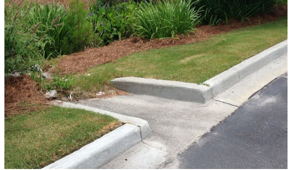
Figure 14. Example of a Concrete Curb with Drainage Opening
