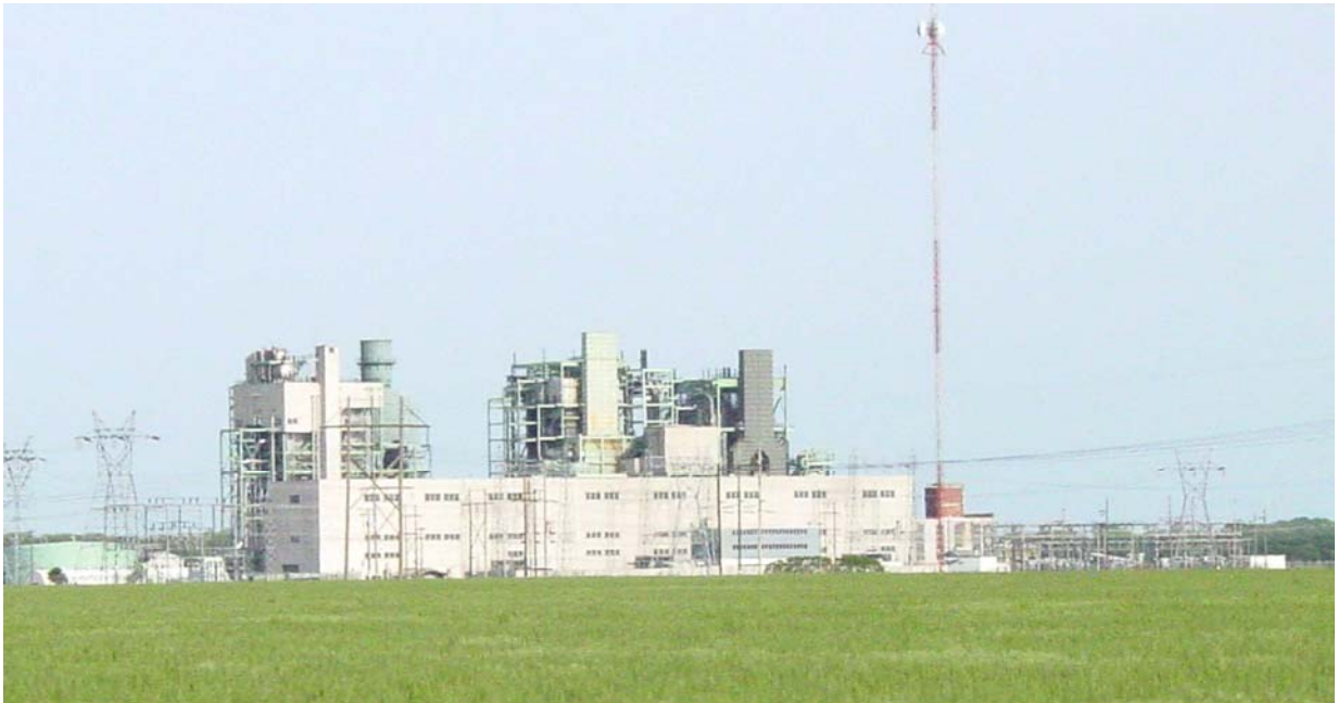
Energy Plant in Southeast Oklahoma County
